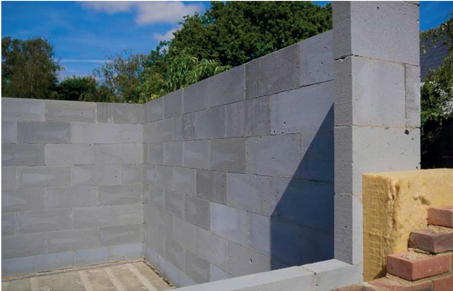
The Thin-Joint, Rå Build method of construction enables a fast, weathertight masonry shell to be built, allowing follow-on trades to start work sooner in a weatherproof environment, whilst retaining the flexibility of on-site construction. Thin-Joint is a recognised Modern Method of Construction and has been fully adopted as the preferred method of wall construction throughout most of northern Europe.
